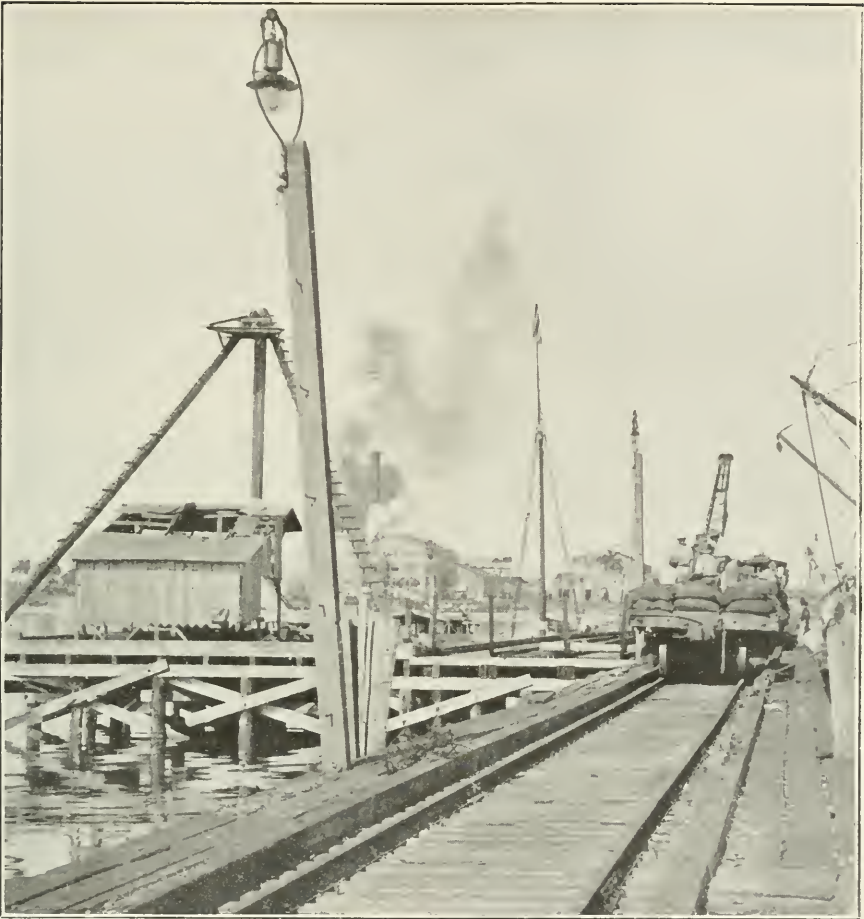
Pier of the Spanish-American Iron Company at Felton, Nipe Bay, Oriente Province. The pier is one-eighth of a mile long, built out far in the bay because of shallow water
