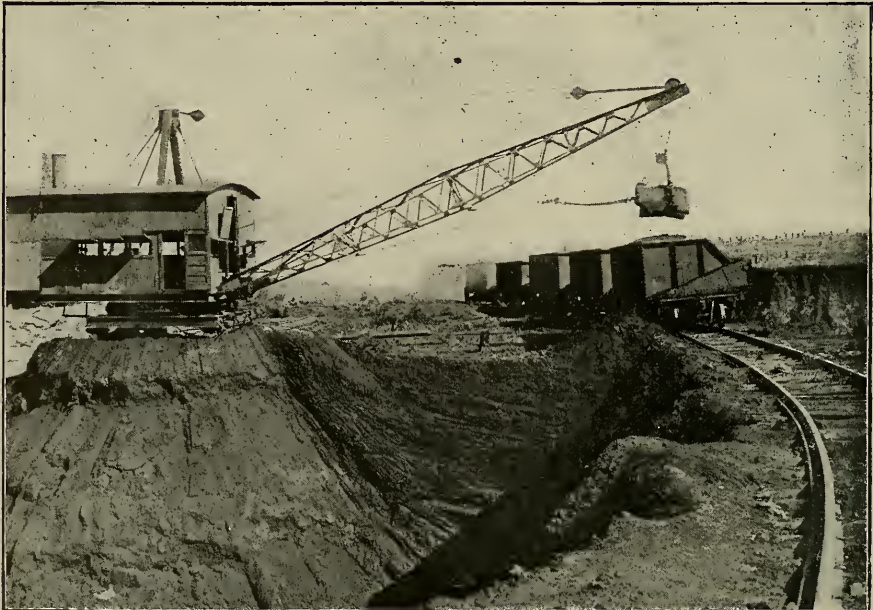
Steam drag at Felton mining properties owned by the Spanish-American Iron Company.
